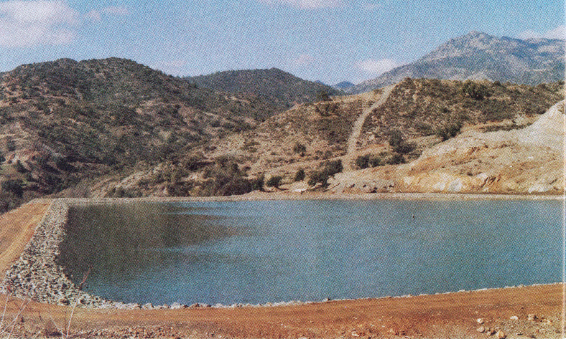
Partial view of Eftagonia No. 1 pond : capacity 92,000 m 3
