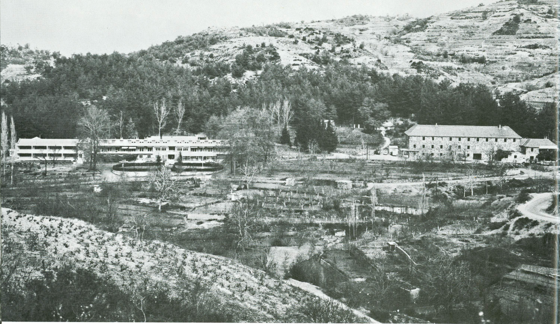
A view of the Kyperounda Sanatorium, which has been converted into a conventional hospital to provide for a 50 bed in-patient facility. A modern surgical theatre and outpatients examination rooms have also been constructed.
