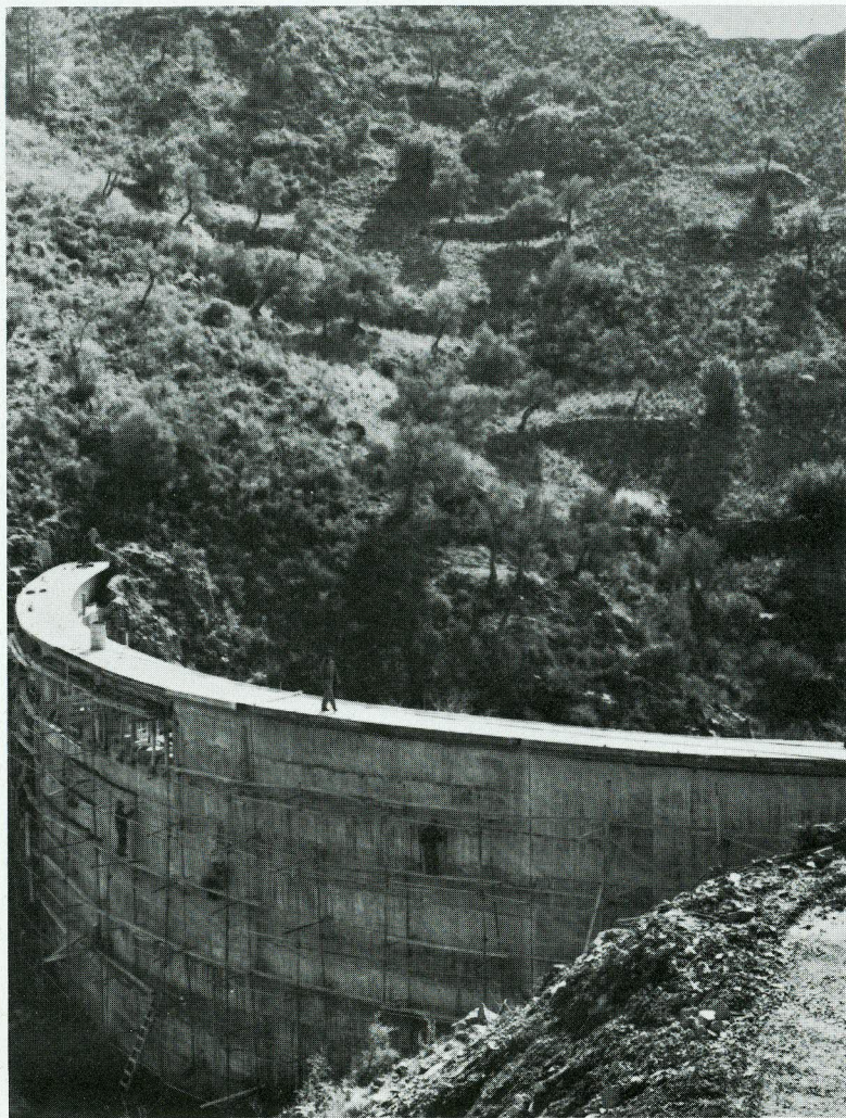
Ayii Vavatsinias arch dam and pond under construction. Both schemes have a total capacity of 108,500 c.m. A joint irrigation distribution system commands an area of 24 hectares.
