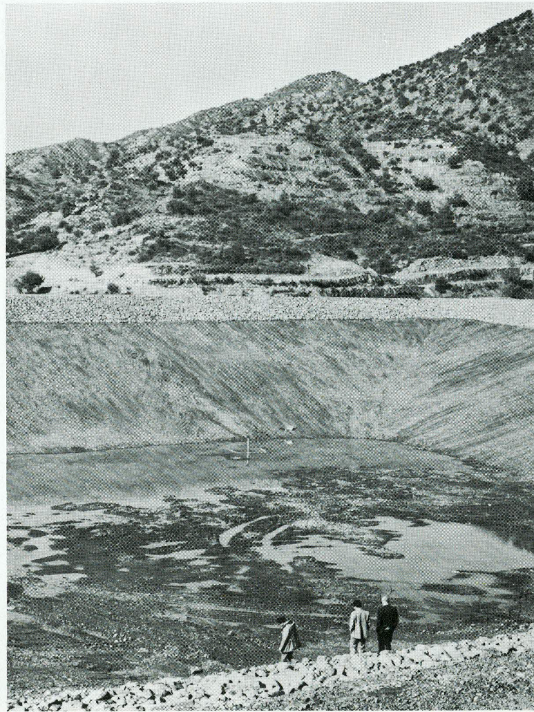
Ayii Vavatsinias arch dam and pond under construction. Both schemes have a total capacity of 108,500 c.m. A joint irrigation distribution system commands an area of 24 hectares.
