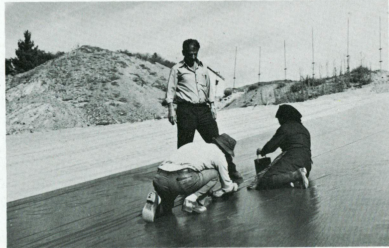
Constructional details at Eftagonia No. I pond (lining of P.V.C. membrane).
