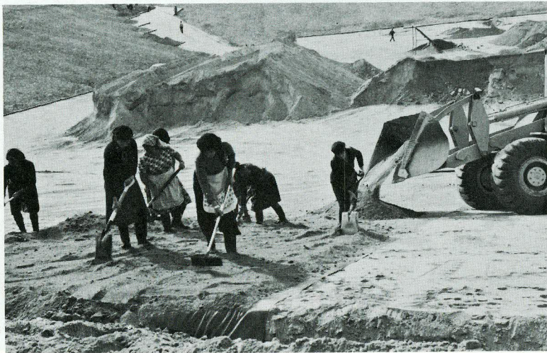
Constructional details at Eftagonia No. I pond (lining of P.V.C. membrane).
